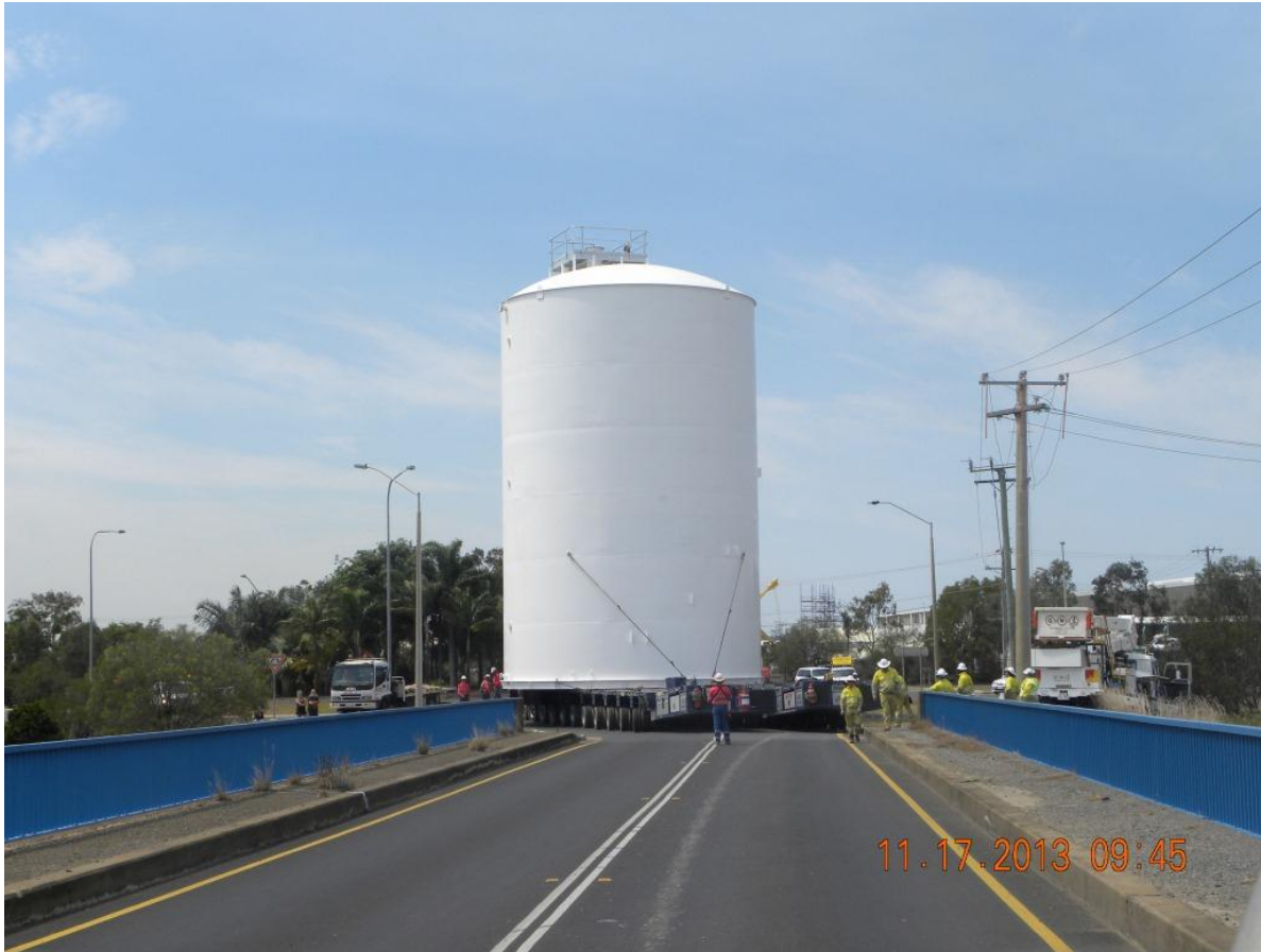
The Raw Water Tank approaching bridge crossing.
