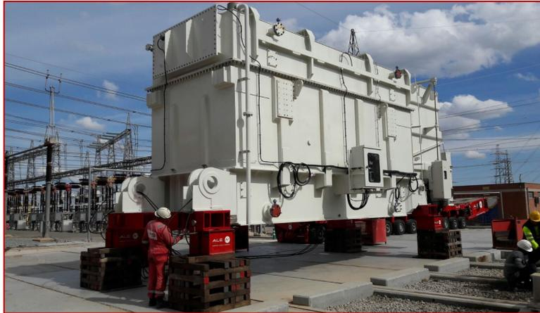
ALE has carried out the replacement of a 205t transformer, located in the work area, with a second 230t transformer, located in the repair area, within the Sentmenat electrical substation.
