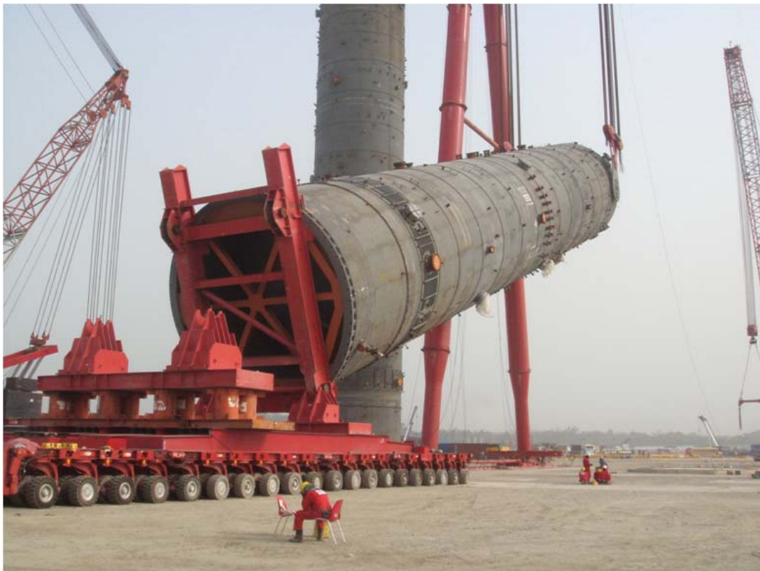
3000t Tailing Frame Capacity 3000 tonnes
