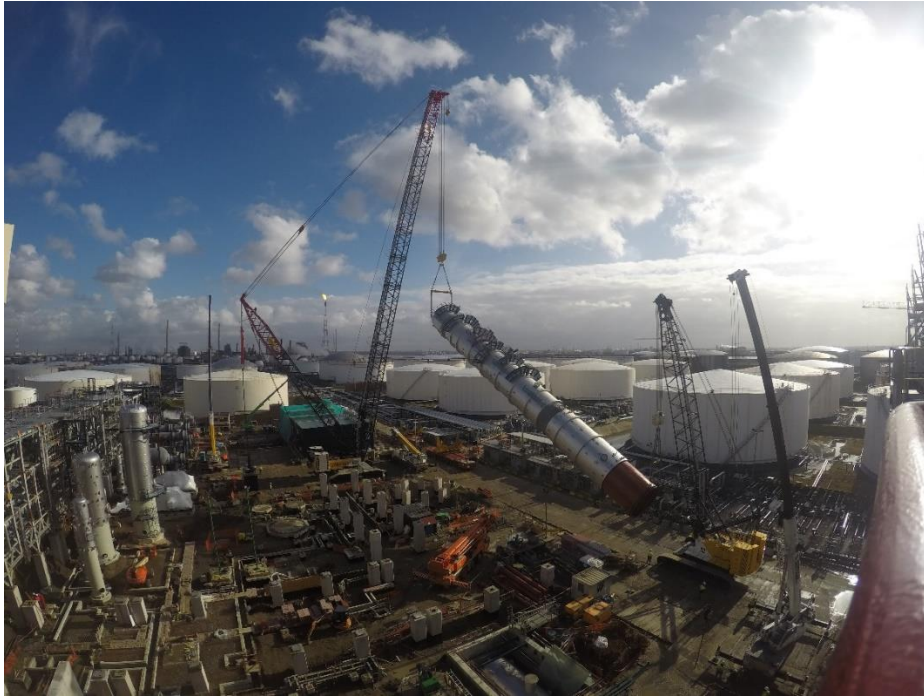
Image 1: Tailing of the main fractionator from horizontal to vertical position.
