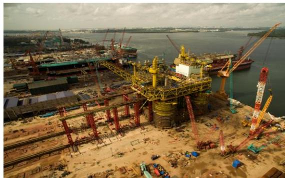
ALE has jacked-up the Malikai Topside 40m high, before skidding the Topside a distance of 90m whilst at this elevation - making these the world's highest jack-up and skidding operations performed on this scale. These operations were carried out whilst executing the Malikai EPC TLP Project at Malaysia Marine and Heavy Engineering (MMHE) West in Johor Darul Takzim, Malaysia.
