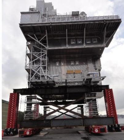
ALE's Mega Jack 800 has been used for the second time in Norway to jack-up a Living Quarter (LQ) module, weighing 2,000t, in November.
