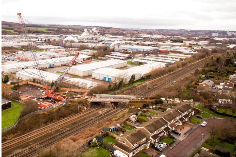
ALE has successfully completed the Chowdene Bank bridge replacement in Gateshead, UK, using the AK912 crane.
