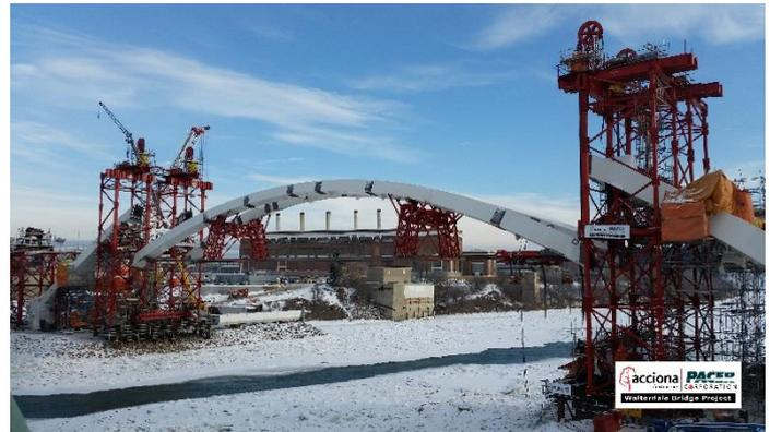
ALE has successfully completed the skidding, navigation and lifting manoeuvres of the 1,000t main arch as part of the Walterdale Bridge replacement project in the city of Edmonton, the capital of Alberta, in Canada.
