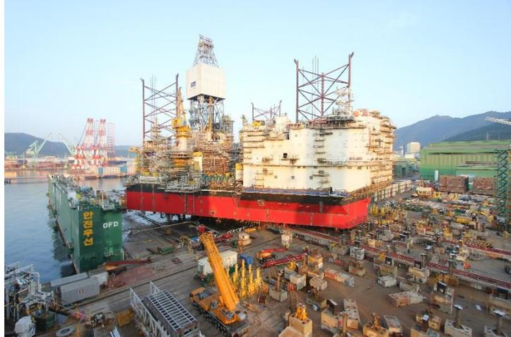
ALE completed the load-out of the 30,000t CAT-J jack-up rig in July, using a unique skidding system especially designed for the project.
