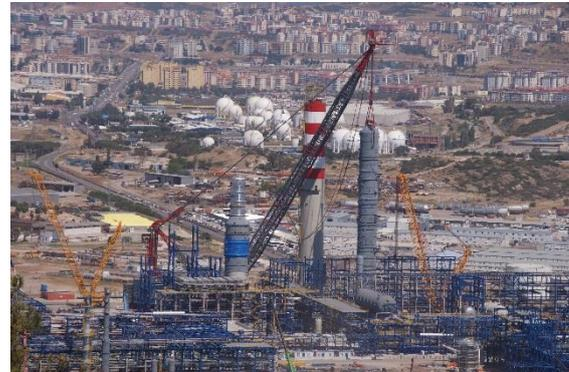
One of the world's largest capacity land based cranes, the AL.SK190, has performed its first lifts in Turkey.
