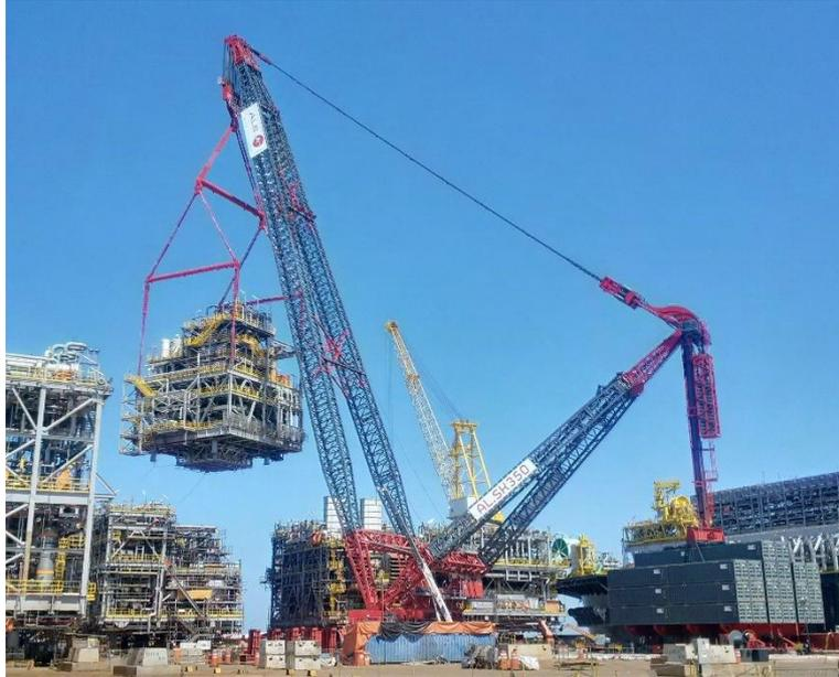
The world's largest capacity land based crane, the AL.SK350, has performed its inaugural lifts in Brazil, using its 4,000t winch system and high speed slew.
