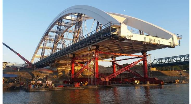
ALE has reached the first project milestone of the Zezelj bridge launch in Novi Sad, Serbia, and has completed the launch of the first section.
