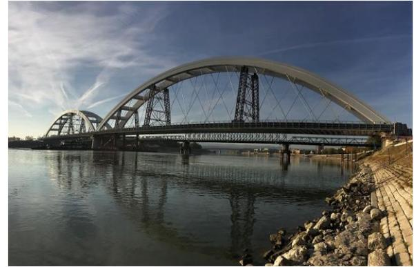
ALE has completed the launching of the Zezelj bridge, weighing 11,100t, in Novi Sad, Serbia, in October 2017.
