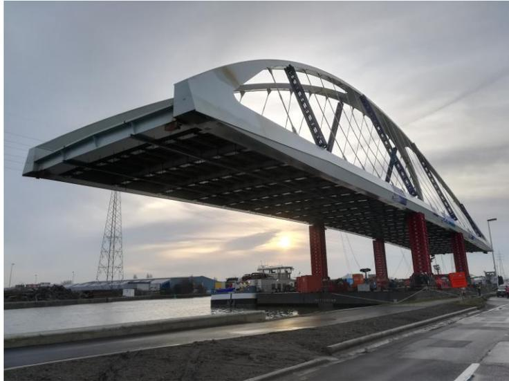
ALE has successfully performed the load-out and installation of a steel bridge using the award-winning Mega Jack 800 in Antwerp, Belgium.
