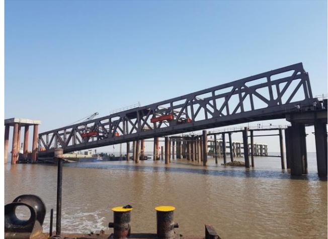
ALE has installed one of the world's longest linkspan bridges using the innovative hydraulic floatover jacks in Gujarat, India.
