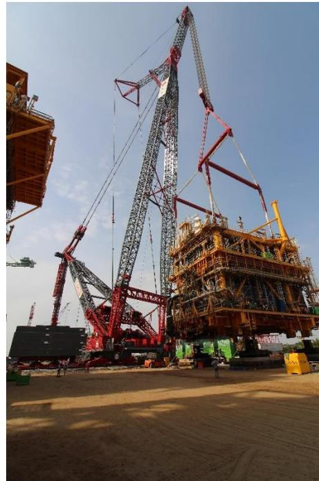
ALE has used its innovative heavy duty jib for the first with the the AL.SK350 crane whilst performing the inaugural lift, weighing 1,276t, of an FPSO module integration project in Nigeria.
