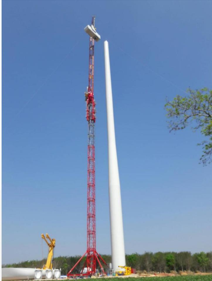
ALE is utilising two innovative tower cranes on Wind Energy Holding's Thepharak wind farm project, Thailand, to handle and install over 700 wind components.
