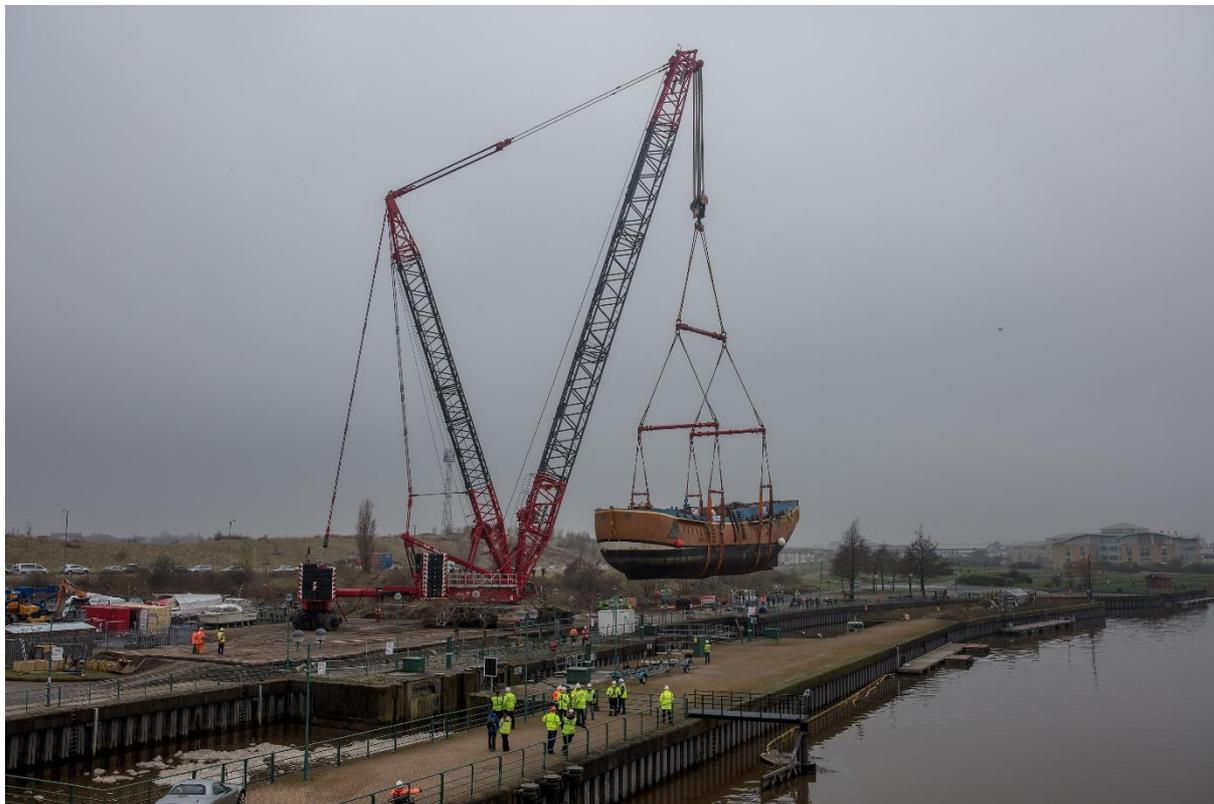
ALE has completed a landmark crane lift of the historic HM Bark Endeavour ship, weighing 274t, in Stockton-on-Tees, UK.
