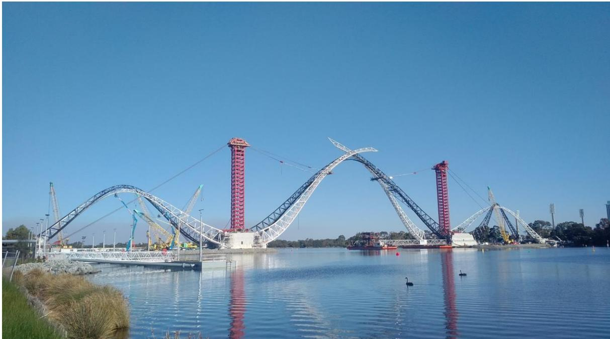
ALE has used its innovative Mega Jack system to lift both halves of the main arch of Matagarup Bridge in Perth, Australia.
