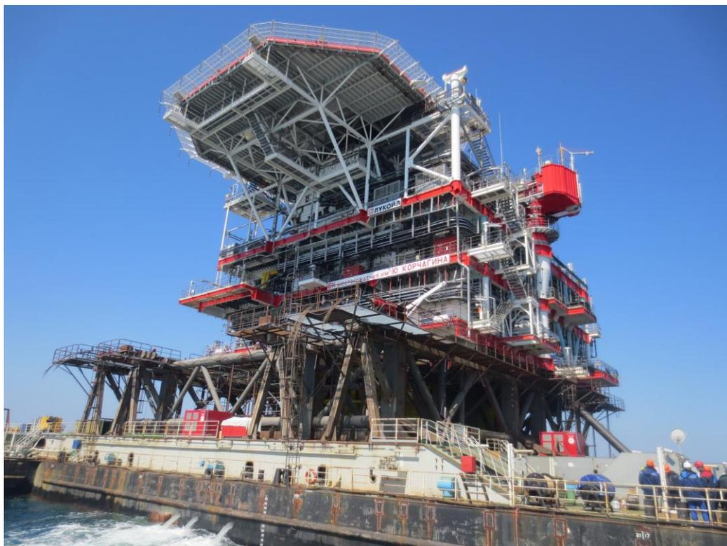
ALE has used a unique offshore skidding technique for the first time to assist with the offshore installation of the satellite platform (SP) topside, weighing 2,565t, for the Korchagin oil field development project in Russia.
