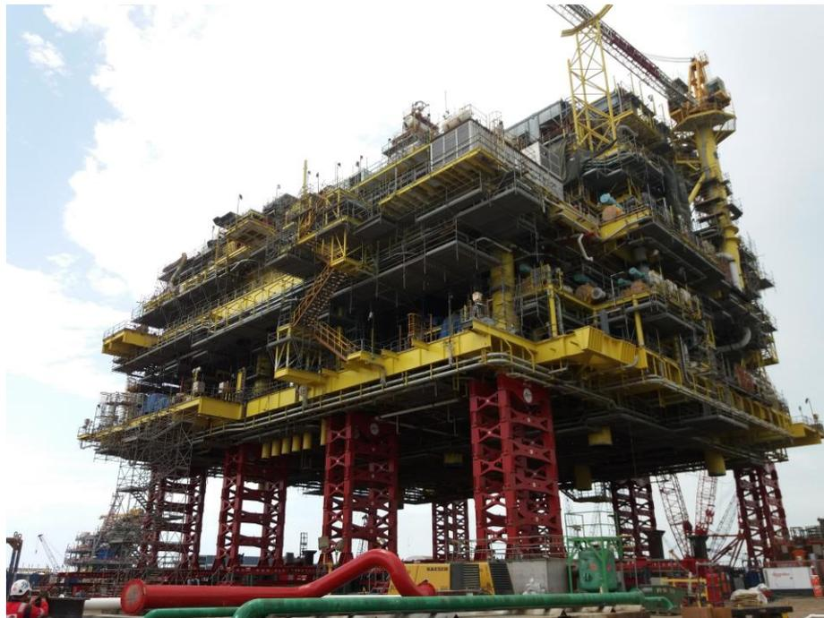
The time and cost efficiency of ALE's Mega Jack system has been demonstrated while completing a 14m-high jack-up of a topside in Mexico.
