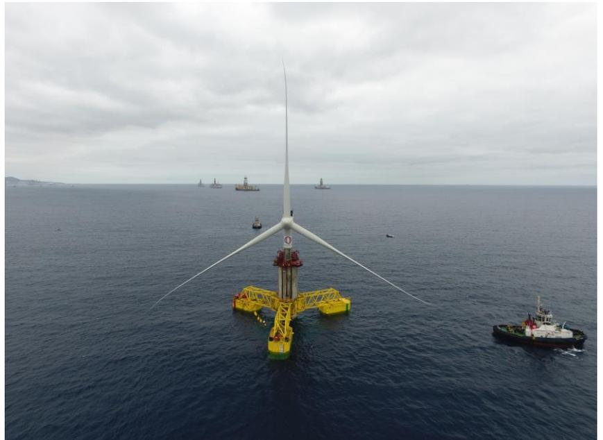
Coordinated by ESTEYCO, the ELICAN project aims to develop a disruptive technology for offshore wind substructures. The concept uses a self-floating GBS and a self-lifting telescopic tower, both made of concrete, which can be fully assembled onshore, turbine included, and conventionally towed to the site.
