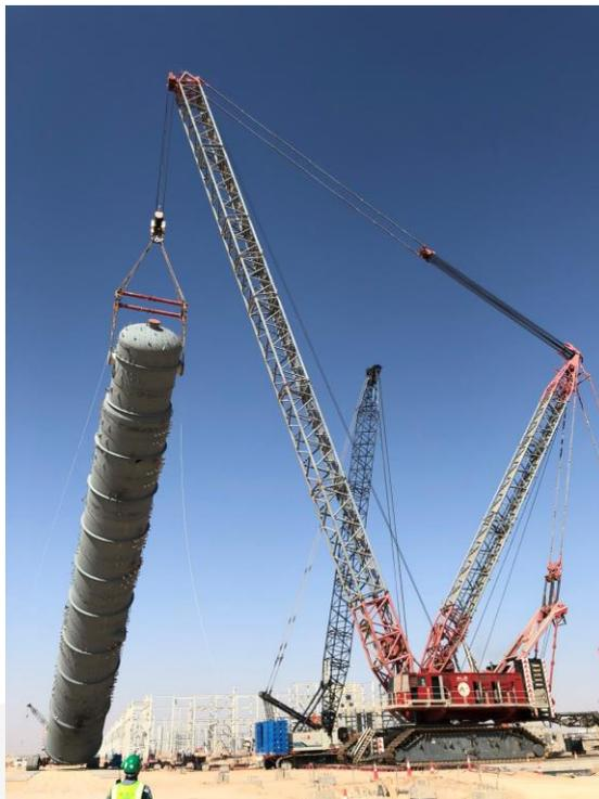
ALE has utilised the largest-ever capacity cranes in Iraq while performing the heavy lifting works at the Karbala Refinery Project. The quick mobilisation of the cranes has also enabled ALE to optimise the overall project schedule.
