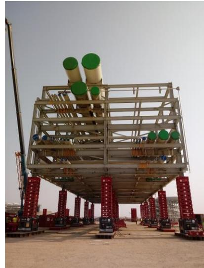
ALE's latest jacking innovation, the Mega Jack 300, has demonstrated its time efficiency, increased stability and ability to work within a restricted project site to jack-up pipe rack modules over 5m high in Kuwait.
