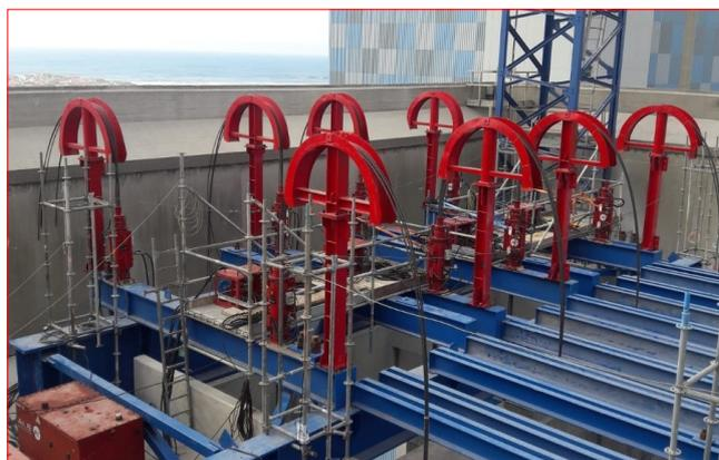
ALE has completed the skidding of a steam drum, weighing 45t, and the skidding and lifting of 8 boiler modules, weighing 50t each, at a paper factory in Figueira da Foz, Portugal.
