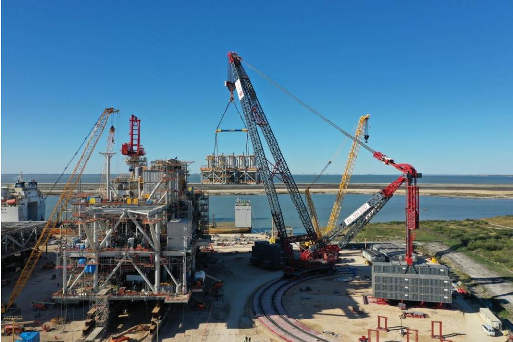
ALE has used the 354,000te/m high capacity and long outreach of the worlds largest capacity land based crane to lift the first of three modules on top of the offshore topside for an oil and gas project in Texas, USA.
