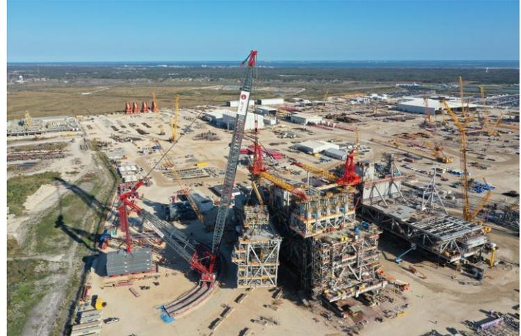
ALE has performed one of North America's heaviest crane lifts using a land based heavy lift crane, lifting the 3179.5 US t (2,884.4 metric tonnes) MRU module, for an oil and gas project in Texas, USA.
