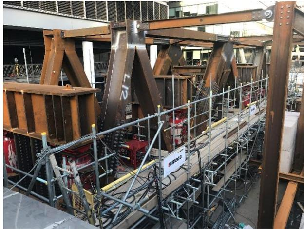
ALE has used its in-house expertise to design, supply, install and perform a bespoke onsite load application, the first load test of its kind in Europe when conducting the progressive loading of a test pile in central London, UK. At 5121t, it was also the highest load test on a pile within Europe.
