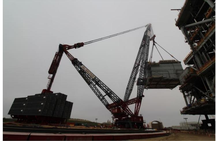
ALE has lifted over 7,000 US tonnes using the world's largest capacity land based crane for an oil and gas project in Texas, USA.
