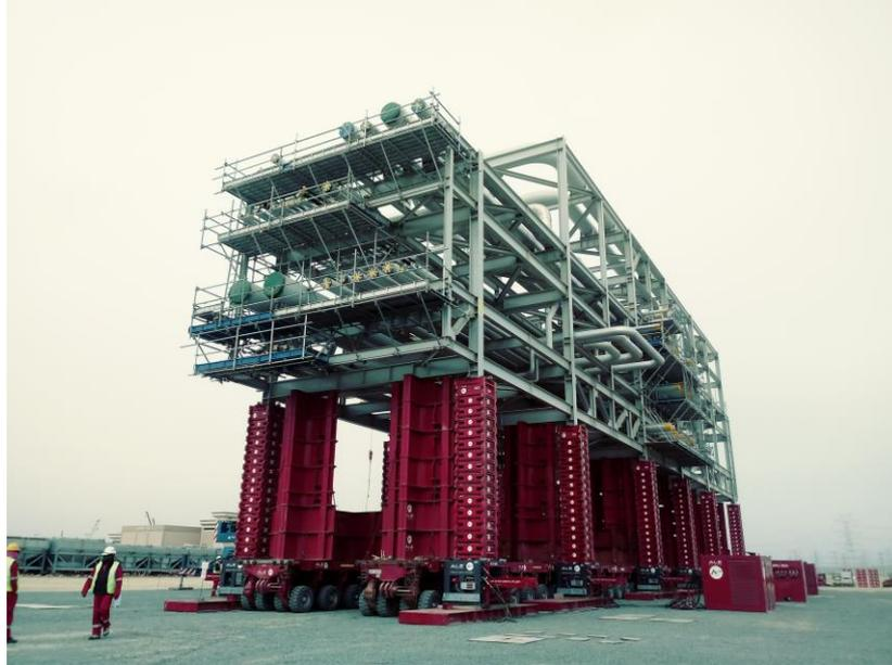
The Mega Jack 300's versatility and efficiency has been demonstrated as it jacked-up, transported and installed a 500t pipe rack module over 7m high in Kuwait.
